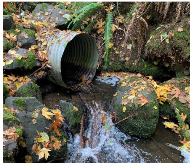
View of existing culvert downstream of 3rd Ave NE
