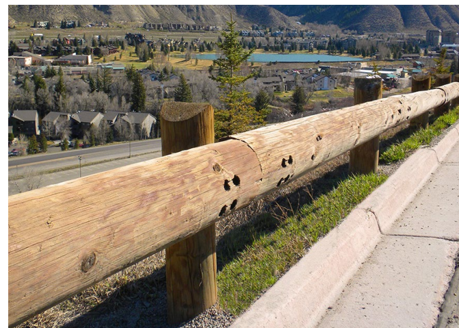
Steel Backed Timber Guard Rail
