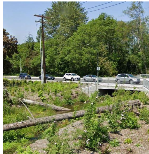
Example of a creek passing through a fish passable culvert with streamside restoration
