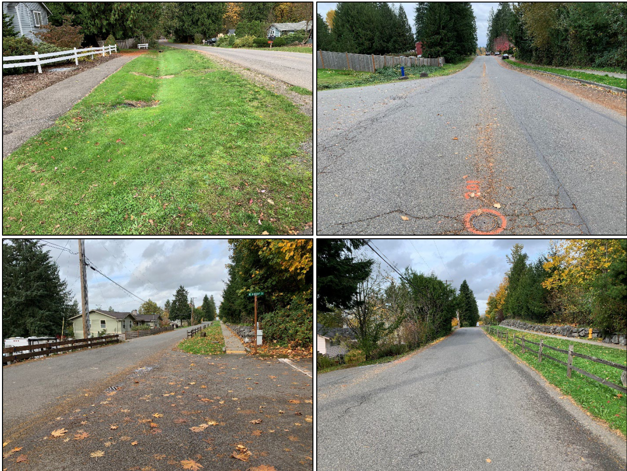
Photos, clockwise from top left: typical roadside grass-lined ditch in southern portion of project; typical roadside conditions with curb on west (right) and ditch on east (left) in southern portion of project; typical roadside conditions without ditches in northern portion of project; typical roadside conditions without ditches in northern portion of project.
