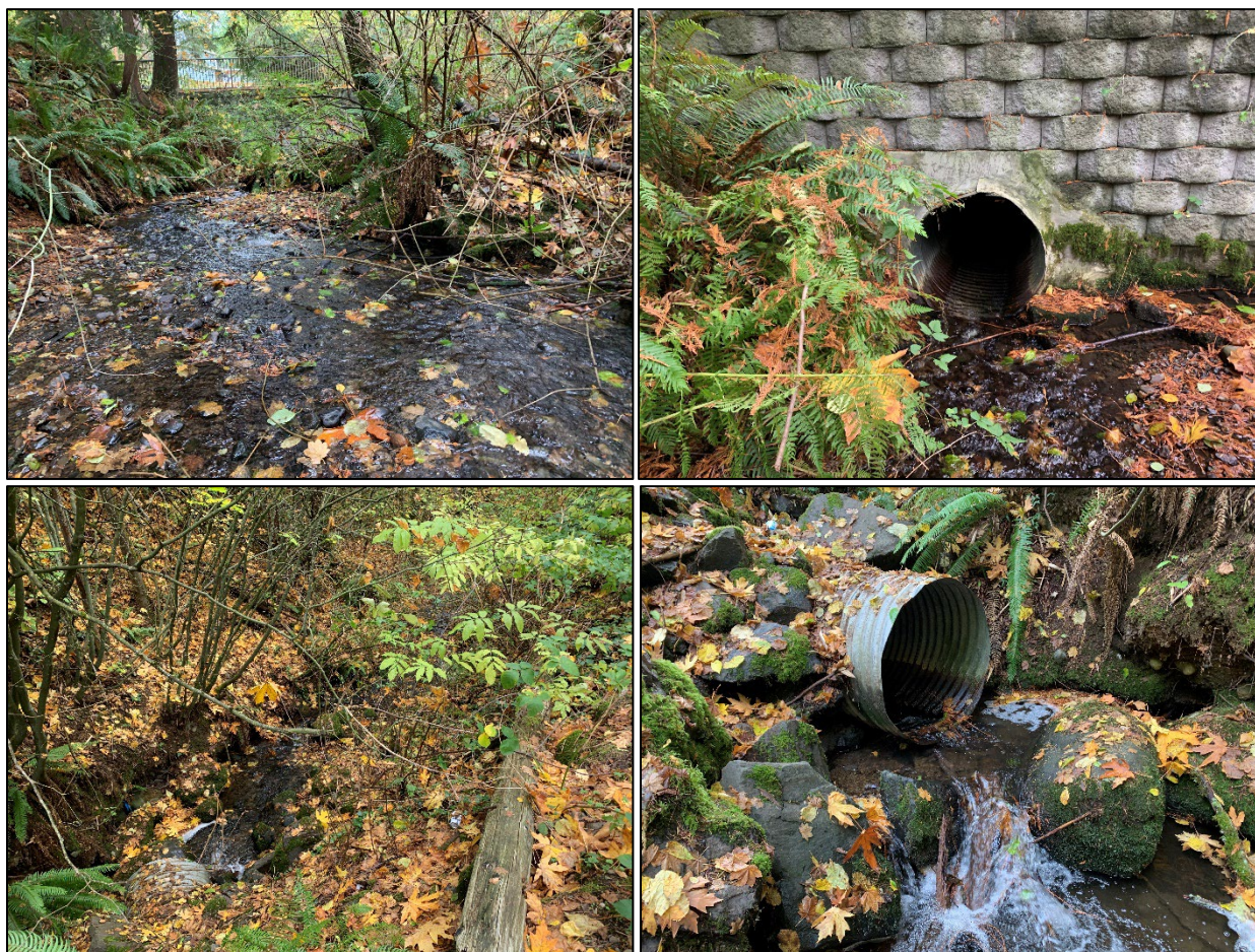
Photos, clockwise from top left: Coe-Clemons Creek upstream of crossing, with 3 rd Avenue road fill prism visible in background; culvert inlet on east (upstream) side of road fill; culvert outlet on west (downstream) side of road fill; Coe-Clemons Creek viewed downstream from roadway.
