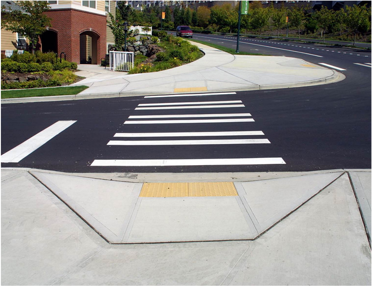
Well-Designed Curb Ramp
