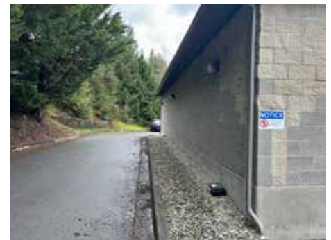
Single point of access to fleet parking
