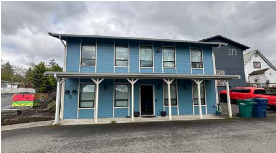
City Hall, west side entrance
