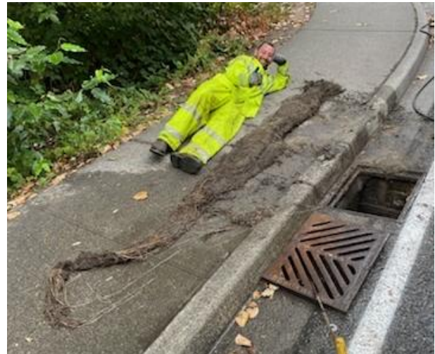
Maintenance crew member poses with giant root ball removed from storm pipe on NE Richardson Street
