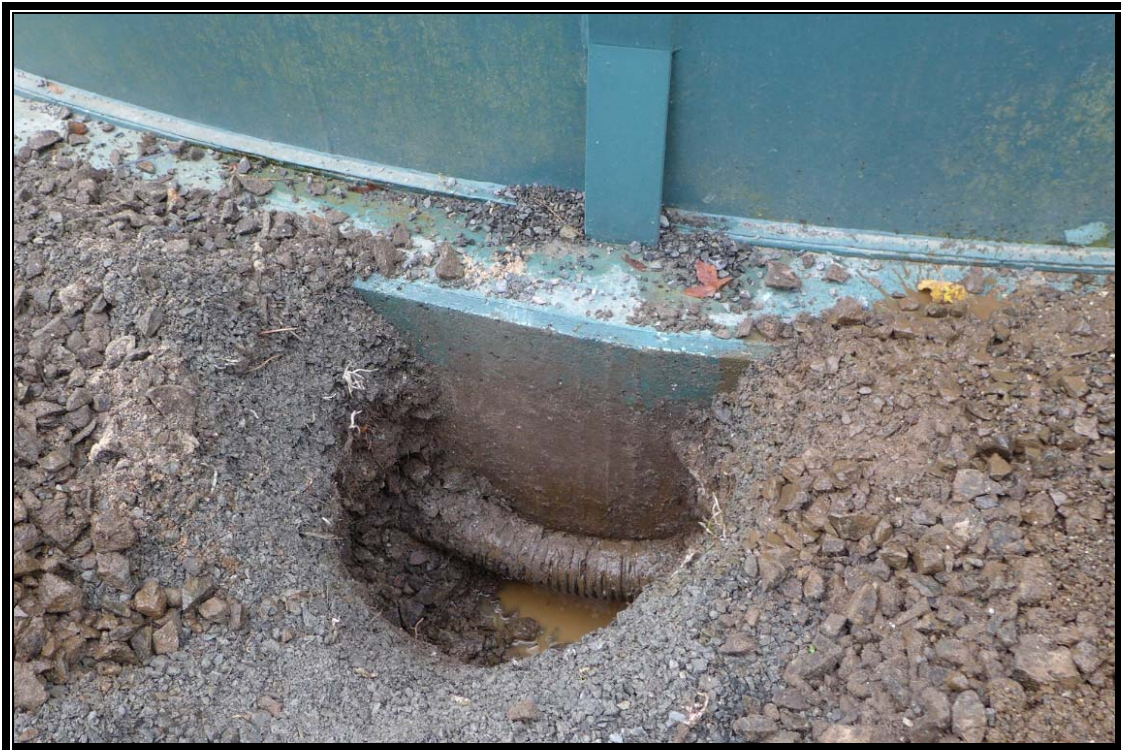
Photograph 8: 0.5MG Reservoir Ringwall Foundation and Drain
