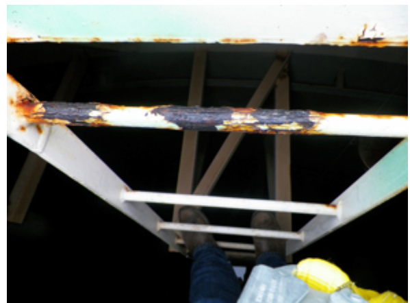
0.5 MG – Interior access ladder
