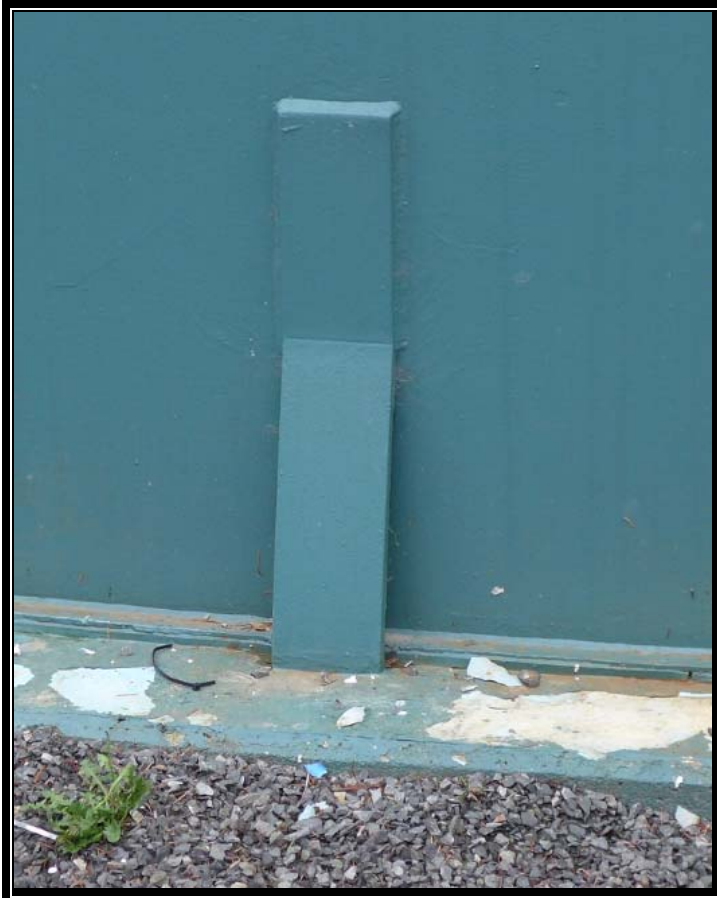
Photograph 3: 0.5MG Reservoir Existing Anchorage
