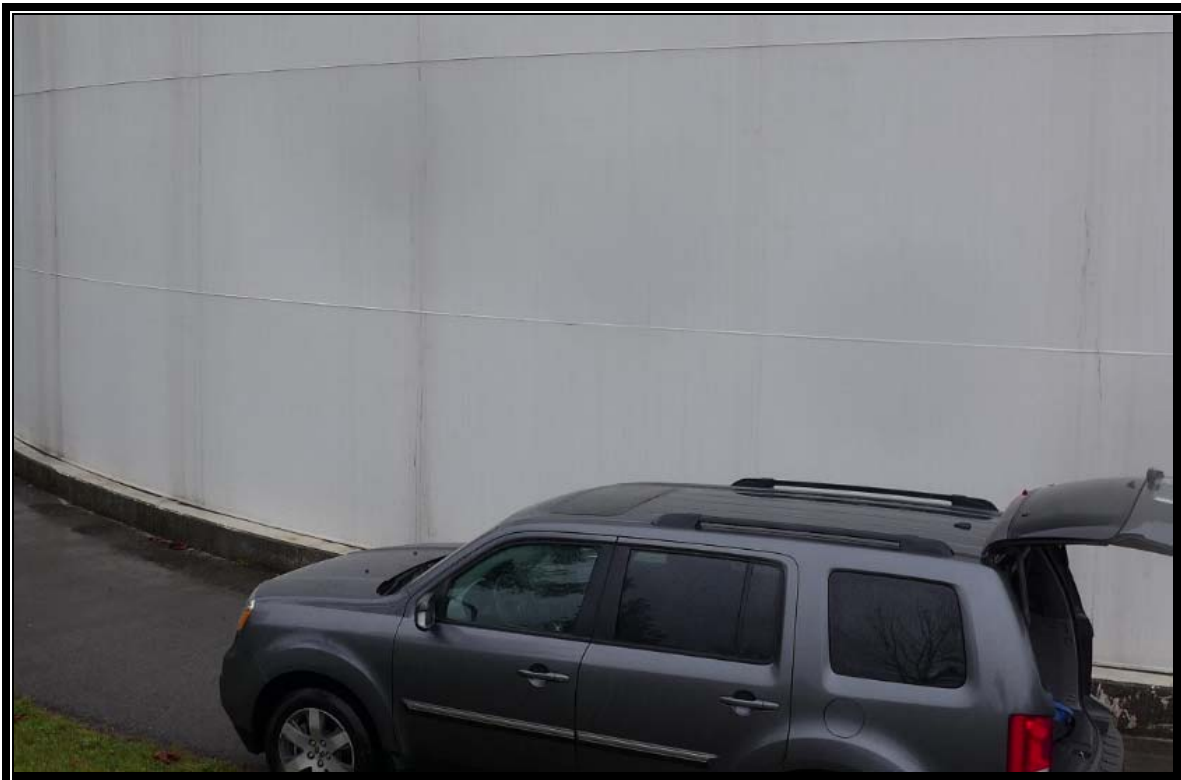
Photograph 14: 2.2MG Reservoir Shell Plates
