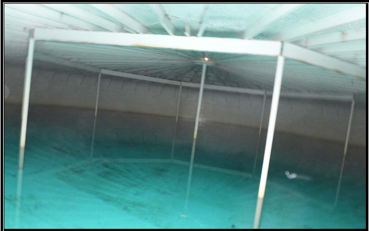
Photograph 17: 2.2MG Reservoir Interior Framing Members
