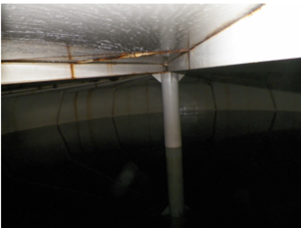
0.5 MG – Roof support beams
