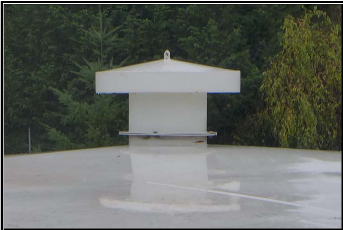
Photograph 12: 2.2MG Reservoir Vent
