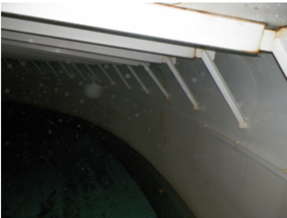
2.2 MG – Interior beam/roof areas
