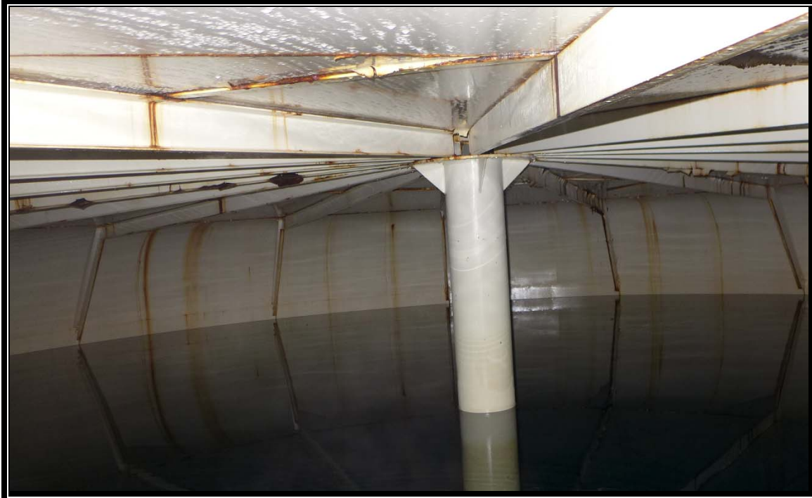
Photograph 9: 0.5MG Reservoir Roof Plates and Supporting Structure
