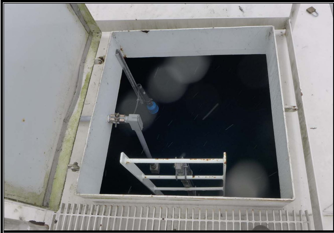
Photograph 11: 2.2MG Reservoir Roof Hatch
