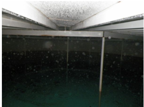
2.2 MG – Interior overview
