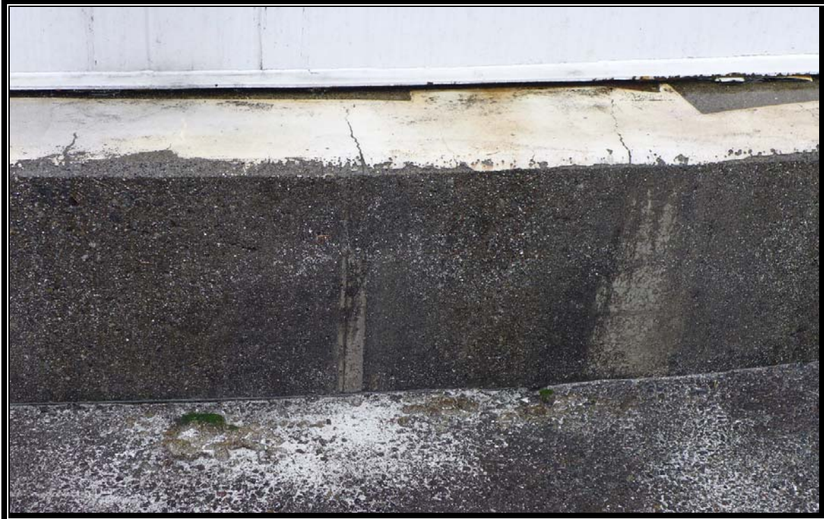
Photograph 15: 2.2MG Reservoir Ringwall Foundation
