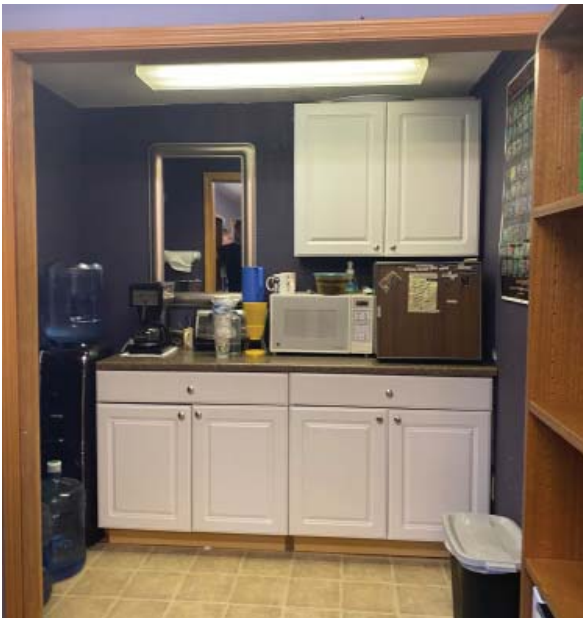
Second floor break area with no existing plumbing.
