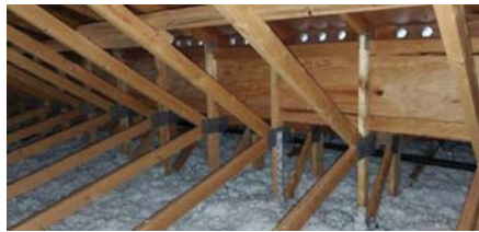
Police Station Roof Structure
