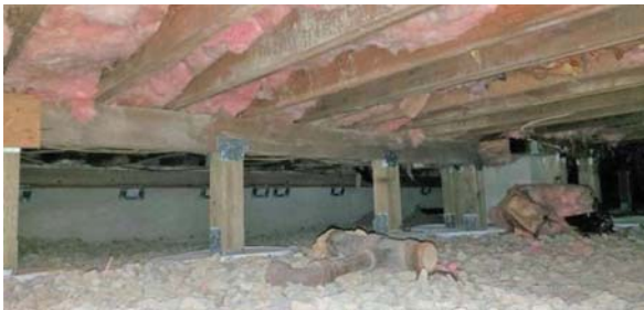
Crawl space anchorage.
