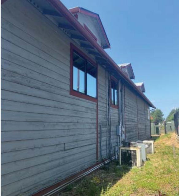
The east elevation faces the public right-of-way on Main Street and features wood siding and dormers.
