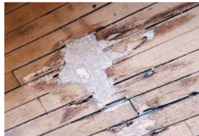
Existing flooring grout repair.
