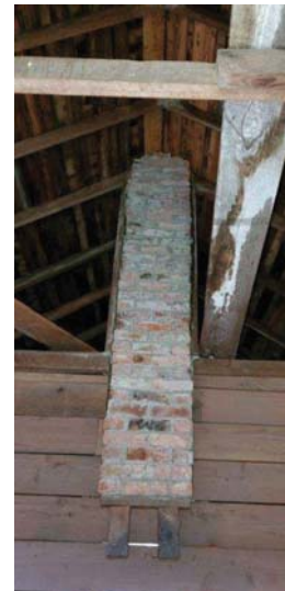
Bunkhouse - Unbraced chimney remnant.
