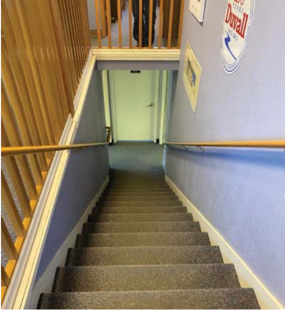
Access to the second floor is by stair only. There are no elevators in the current facility.
