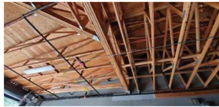
Sally Port Roof Structure
