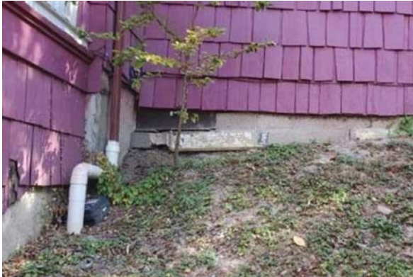
West foundation wall at the south wing
