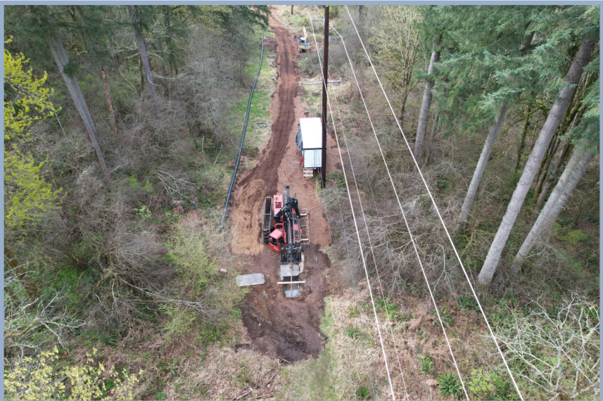
Tolt 2 Transmission Line Replacement construction project
