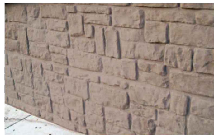
DETAIL 3 - STRUCTURAL EARTH WALL FINISH NTS
